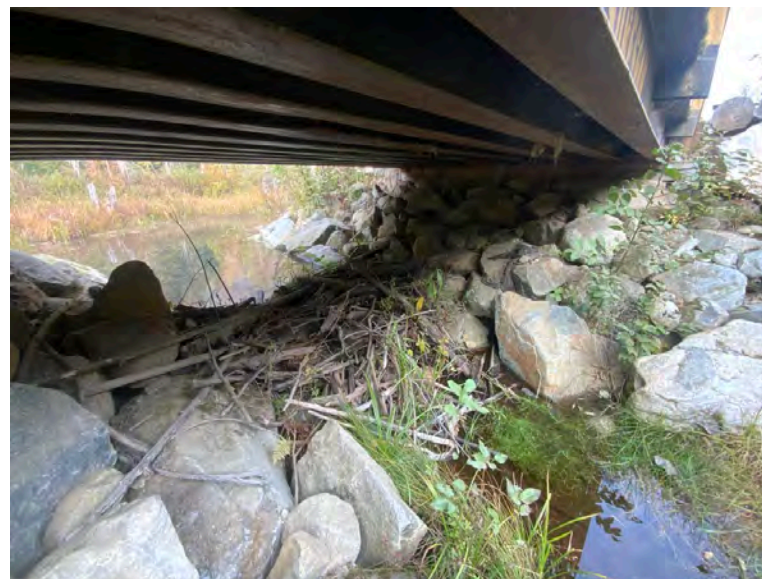
Left Bank Abutment when facing downstream
