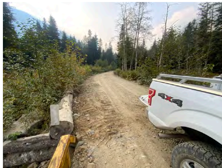
Approach from Right Bank when facing downstream
