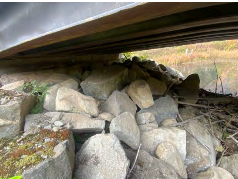
Right Bank Abutment when facing downstream
